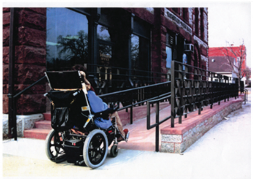
Ramp to general office, restaurant and council meeting and conference doors.
